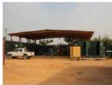
Warehouses and fabshop
